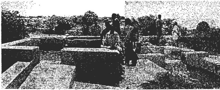
Typical stilling basin structures
