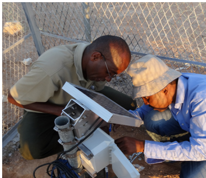
Groundwater level monitoring equipment installation in Garowe
