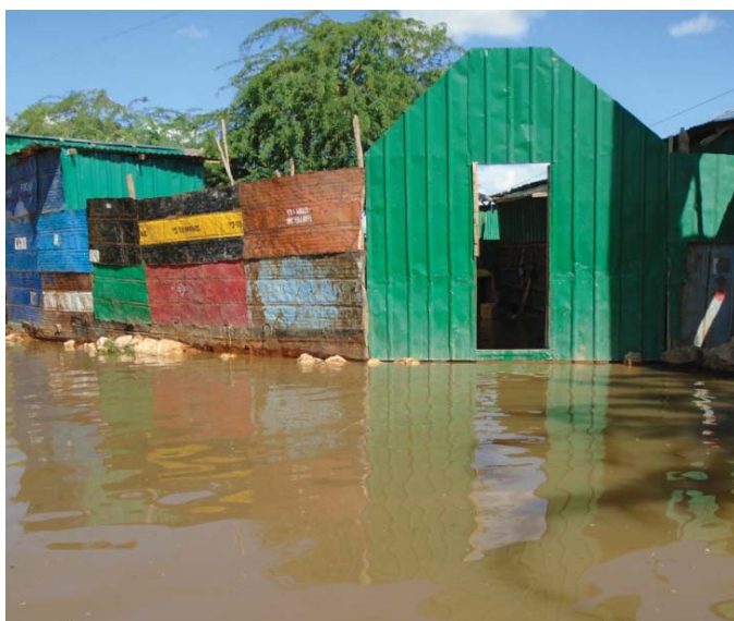
Flooded business property in Belet Weyne during Deyr 2014 rainy season
