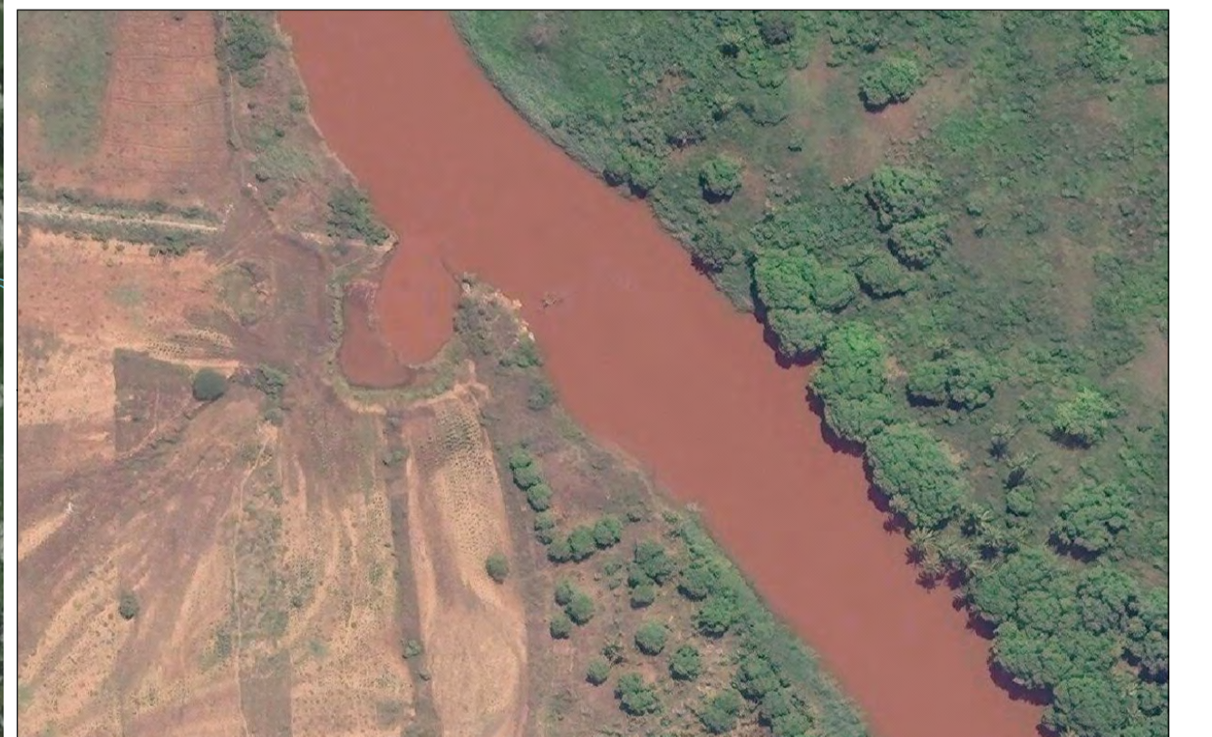
Mashaaga (25 Jun 15) - The river bank is broken at this point with water spilling out probably to irrigate the nearby farm land.
