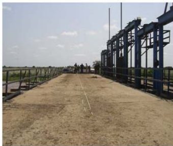
The Barrage deck slab in relatively good condition
