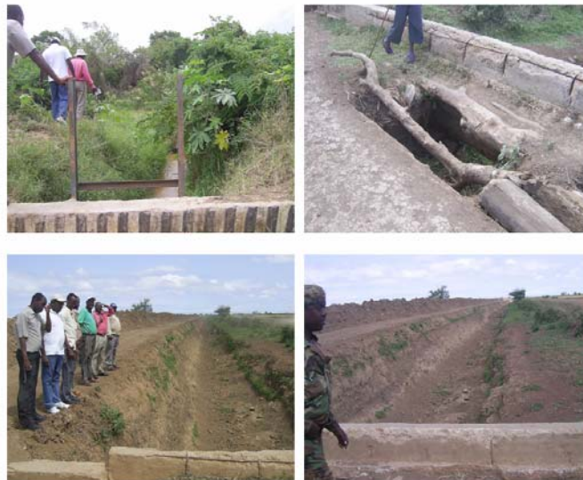
Figure 6.8: Status of primary canals taking off Falkerow barrage 5
