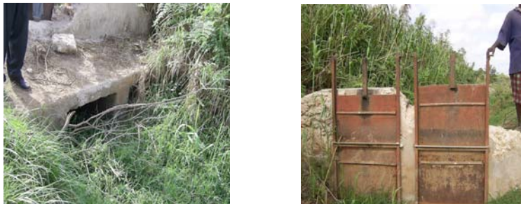
Figure 6.2: Status of some of the canals taking off Genale barrages 4
