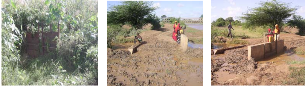
Figure 6.6: Status of some of the primary canals in Qoryooley barrage area
