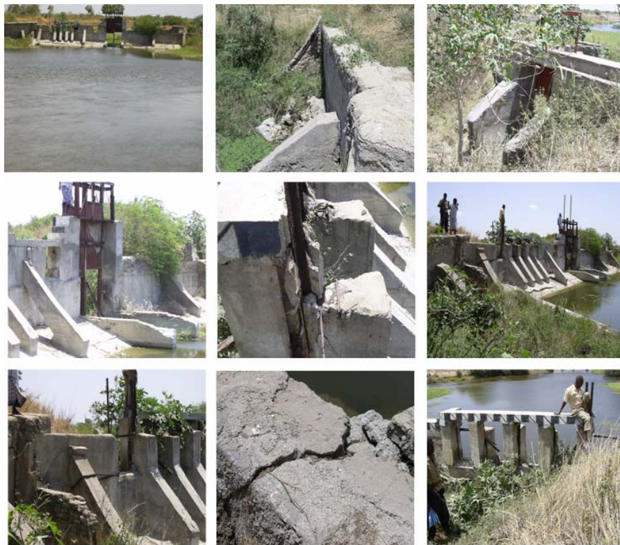
Figure 6.12: Current status of Haway barrage and its canalization system
