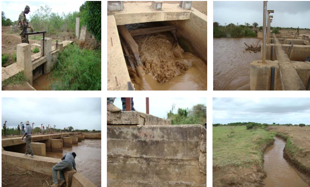
Figure 6.1: Photos showing the current status of Sabuun barrage
