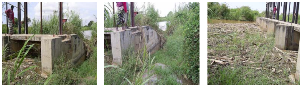
Figure 6.3: Current status of Mashalay barrage
