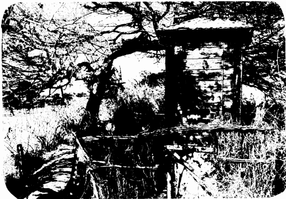
JAMAAME - ( 25.3.80 ) - Looking upstream along the left bank at the Recorder House and well. The 'MP' Point is at the door (top of the concrete ring, a small arrow mark chipped into the concrete, with an R.L. value of 96.97 m.)
