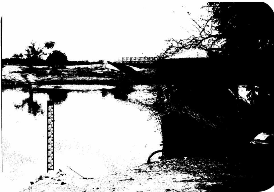
BARDHEERE - (24.3.80) - Looking from the left bank near the Recorder House to the right bank bridge abutment. 4-6 meter gauge on left. This gauge accepted as the reference point for the replacement of the other gauges. There is a TBM on corner of concrete trough nearest the Recorder House (R,L. 100.793 m).
