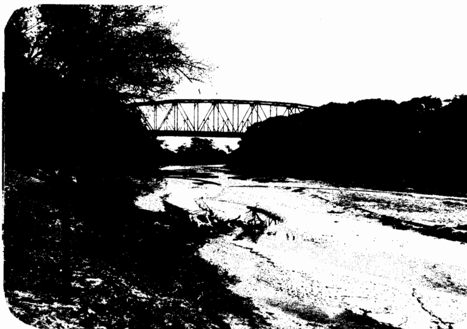
JAMAAME - ( 25.3.81 ) - Looking downstream from the gauging station on the left bank. The bridge is approximately 150 meters D/S of the station. Note that the river bed is lower than the Gauge Zero. The gauge visible in the picture is the 0-2 meter stand, which is partially silted up.
